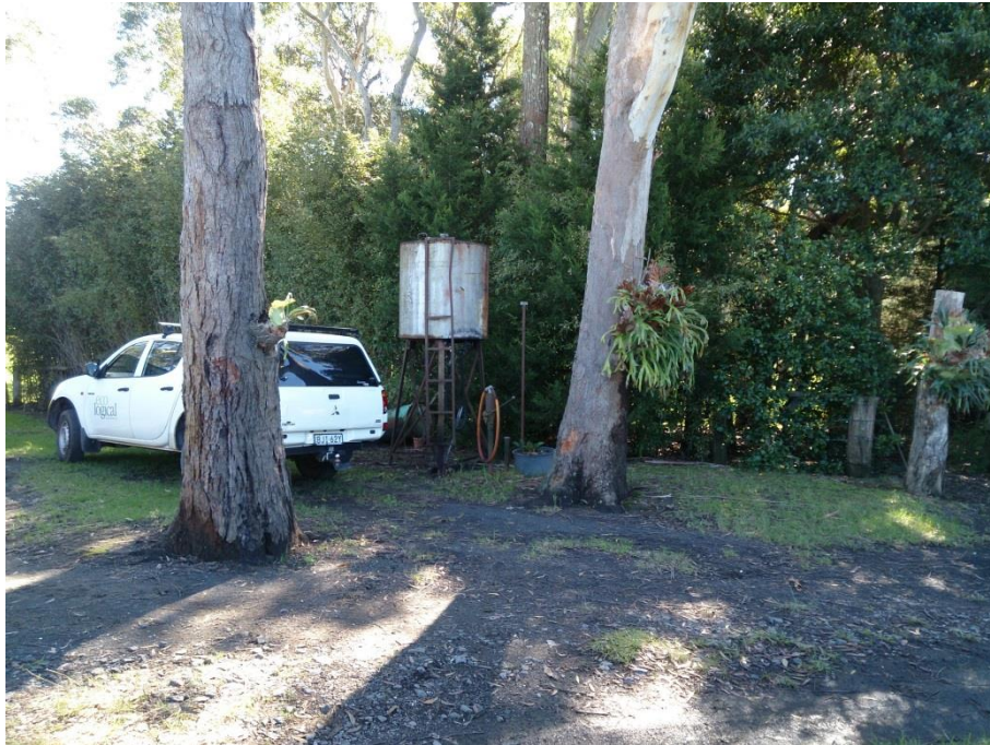
Figure 5 – Raised diesel tank. Older, buried, tank is beneath
