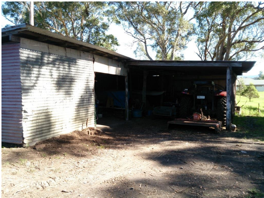
Figure 6 – Western Machinery Shed
